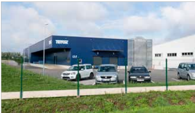
7. 12. In 2021, a new hall with a usable area of almost 3,000 m 2 was approved.
